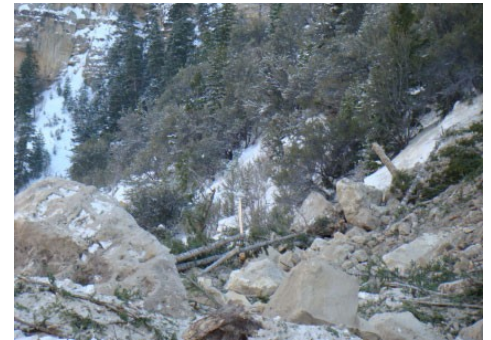
Another view of the landslide area on Highway 14
